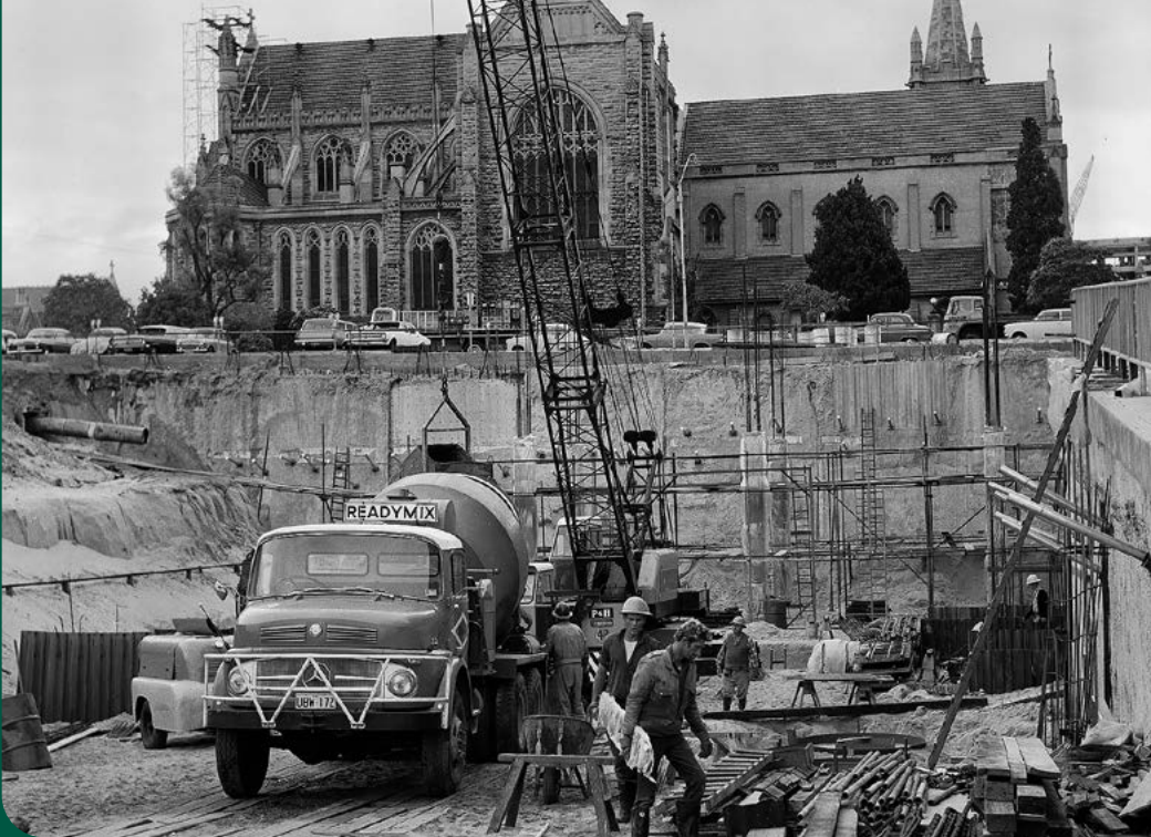
Above: External foundations for extensions to South-East Wing and site for new steam plant - old intersection of Victoria Square and Lord Street.
